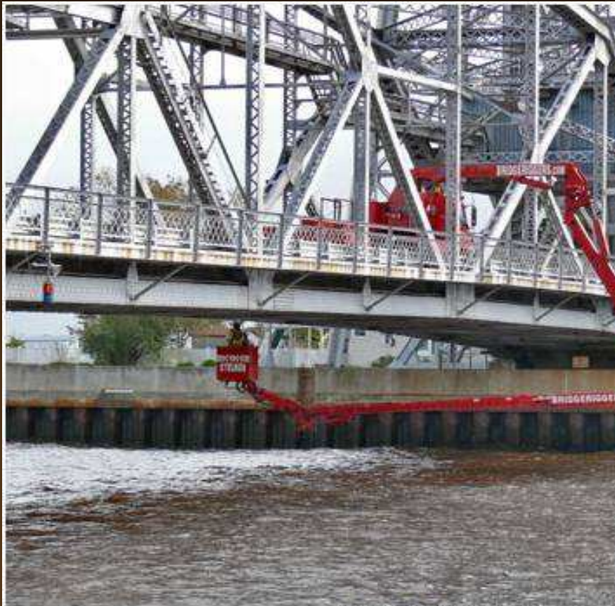
Snooper truck inspection. Photo courtesy of Duluth Shipping News.
